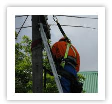
addition of a front and back lanyard and allows you to move your working position while remaining attached to the structure. It keeps you upright if you fall and is more comfortable. When climbing on structures where free-fall is possible, lanyards must be attached to fall-arrest rated anchor points. A lanyard should limit your fall to set standards determined by EEA. This is generally 600 millimetres or less.
